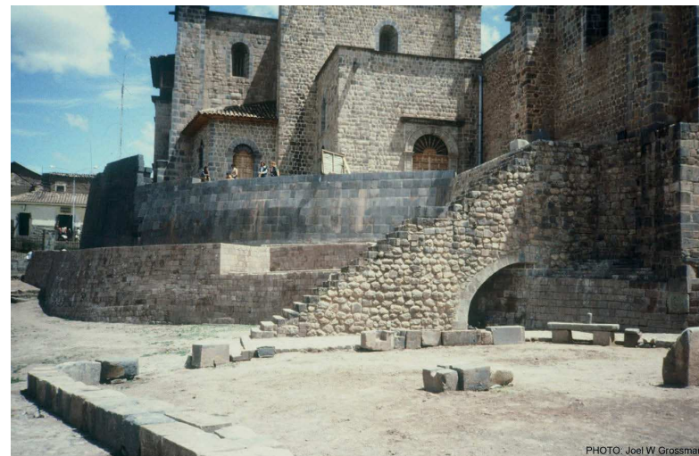
Plate 7a. The Spanish Church of Santo Domingo built atop the curved finely cut stone wall of the Late Horizon Inca temple of Coricancha in Cuzco (Photo by Joel W. Grossman).
